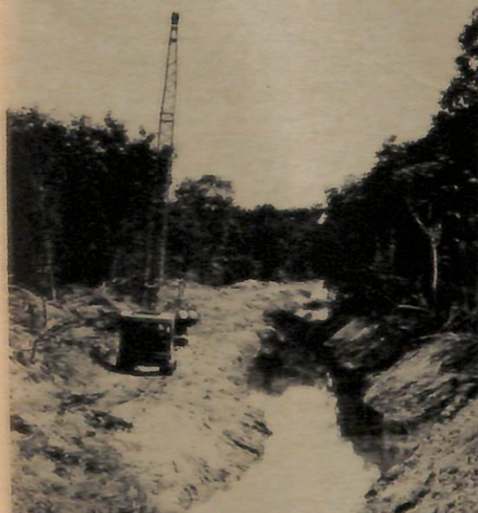
WORK is currently in progress on a project to improve the drainage system along Jalan Berakas.
