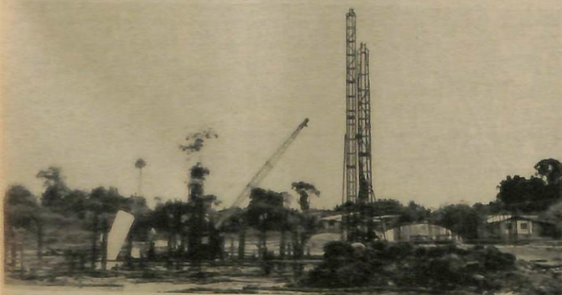
With site clearing works completed, actual construction of the Welfare Home begins as this picture shows.
